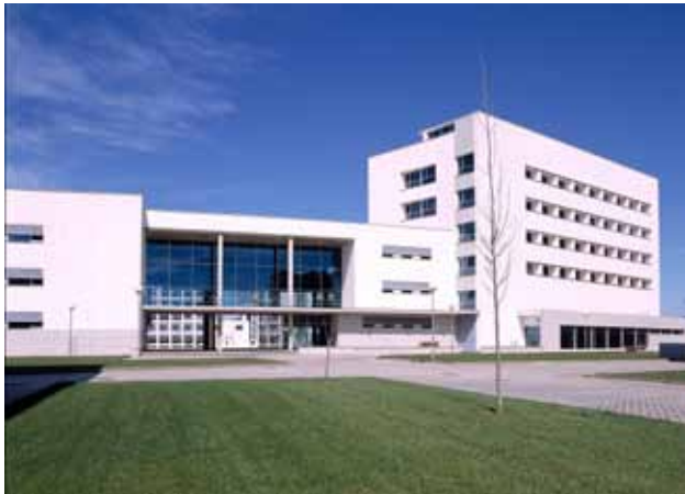
Front view of the congress building
